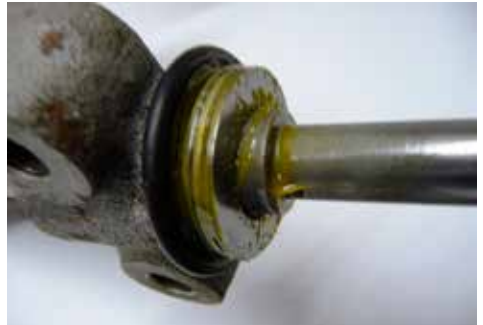
Trunnion removed after grease injection
