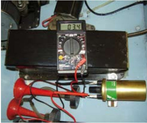
Checking low tension
