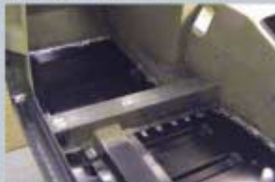
▲ The strength of the shell comes from the floor and pillars, so Dave braced the door apertures and honed his welding skills, replacing everything involved.
