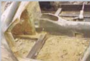
▲ The floor was in a particularly bad way. Having been neglected for so long, it was the usual story of the bottom three inches of the car being non-existent.
